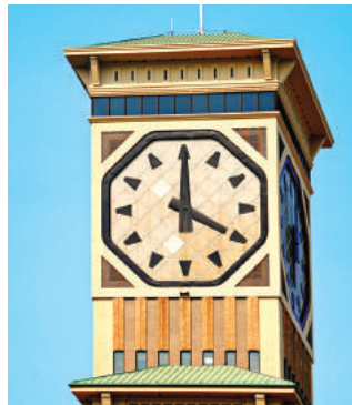
Allen-Bradley Clock Tower, the USA
